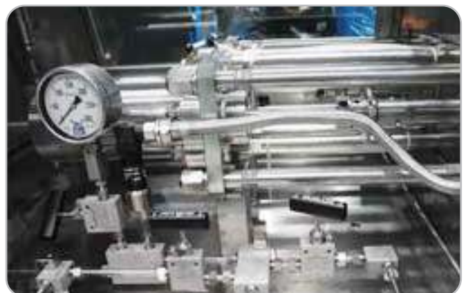
Cooling line on the high pressure part
